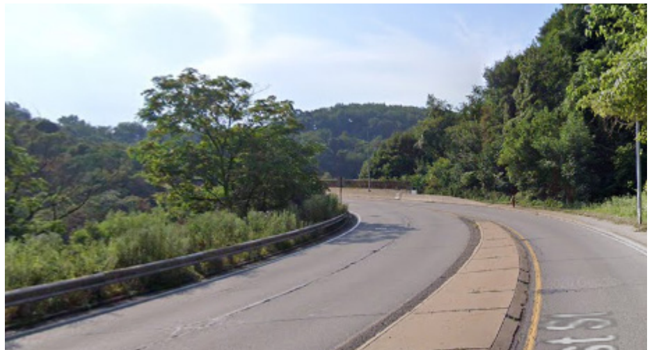
Existing Conditions at East Street near Venture Street
