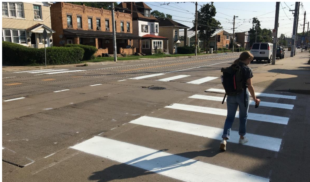
New Crosswalks, July 25, 2019
