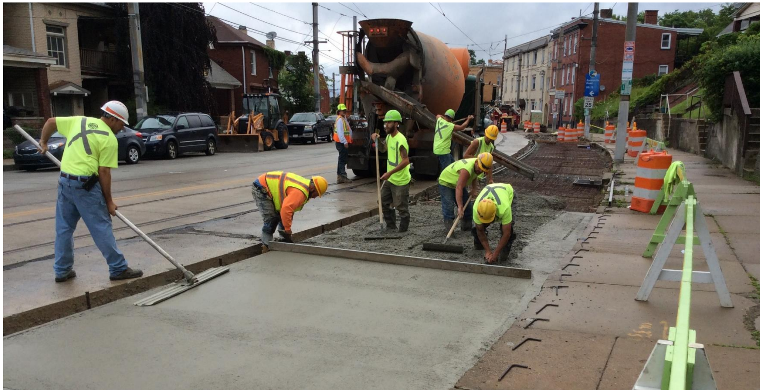
New Concrete, June 21 2019
