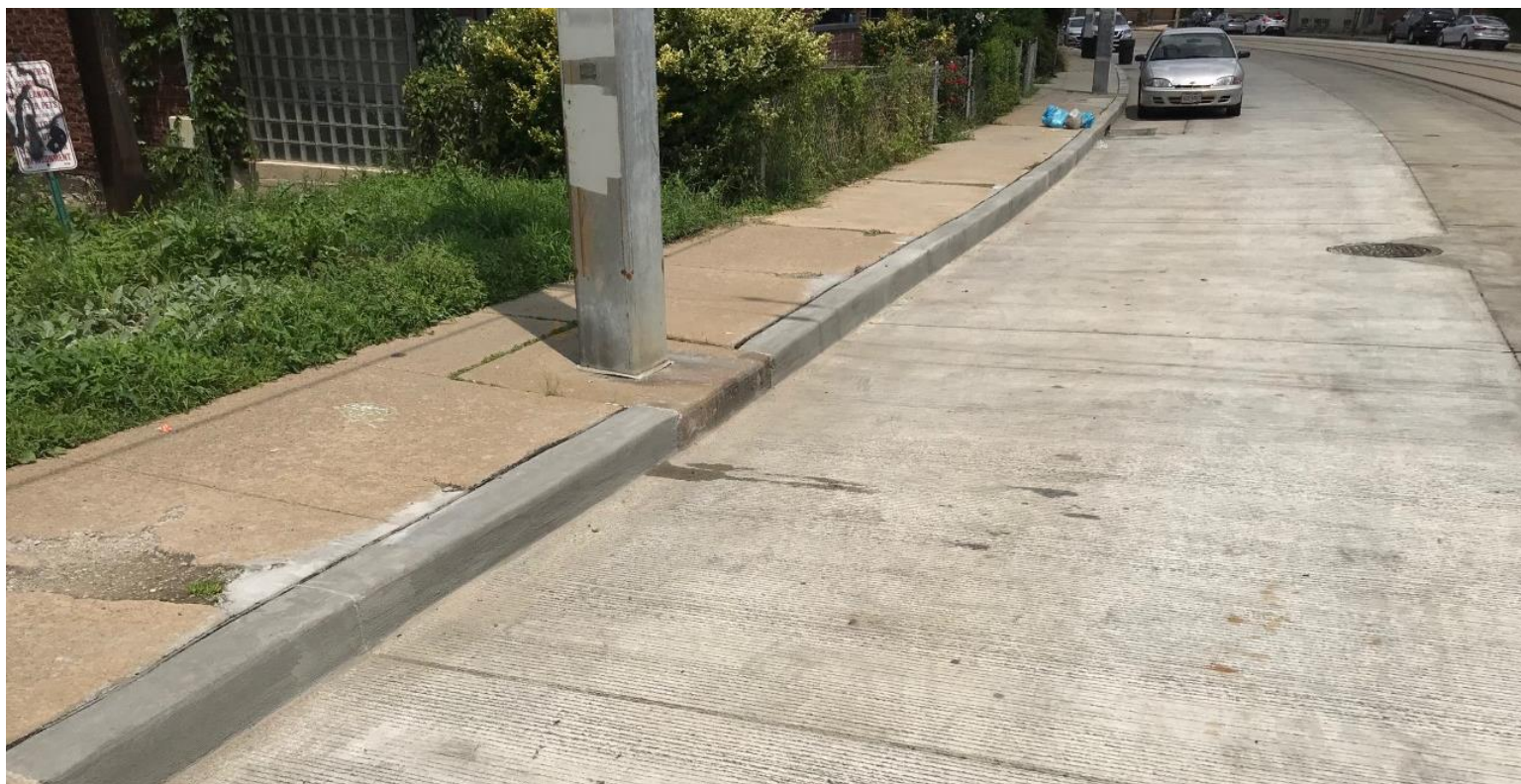
New Concrete, July 10 2019
