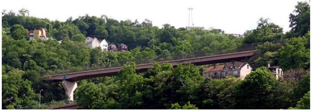
McArdle Roadway Bridge over E Sycamore St
