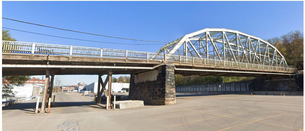
28 th Street Bridge – Originally constructed in 1931
